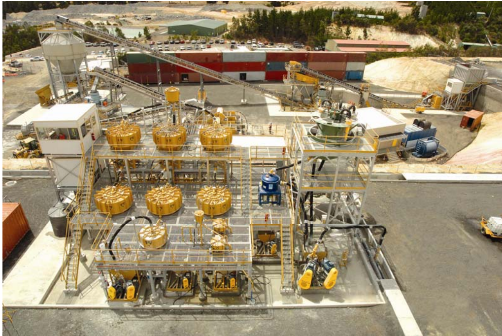
Figure 6: The complete gold processing plant - designed and installed by Gekko.
